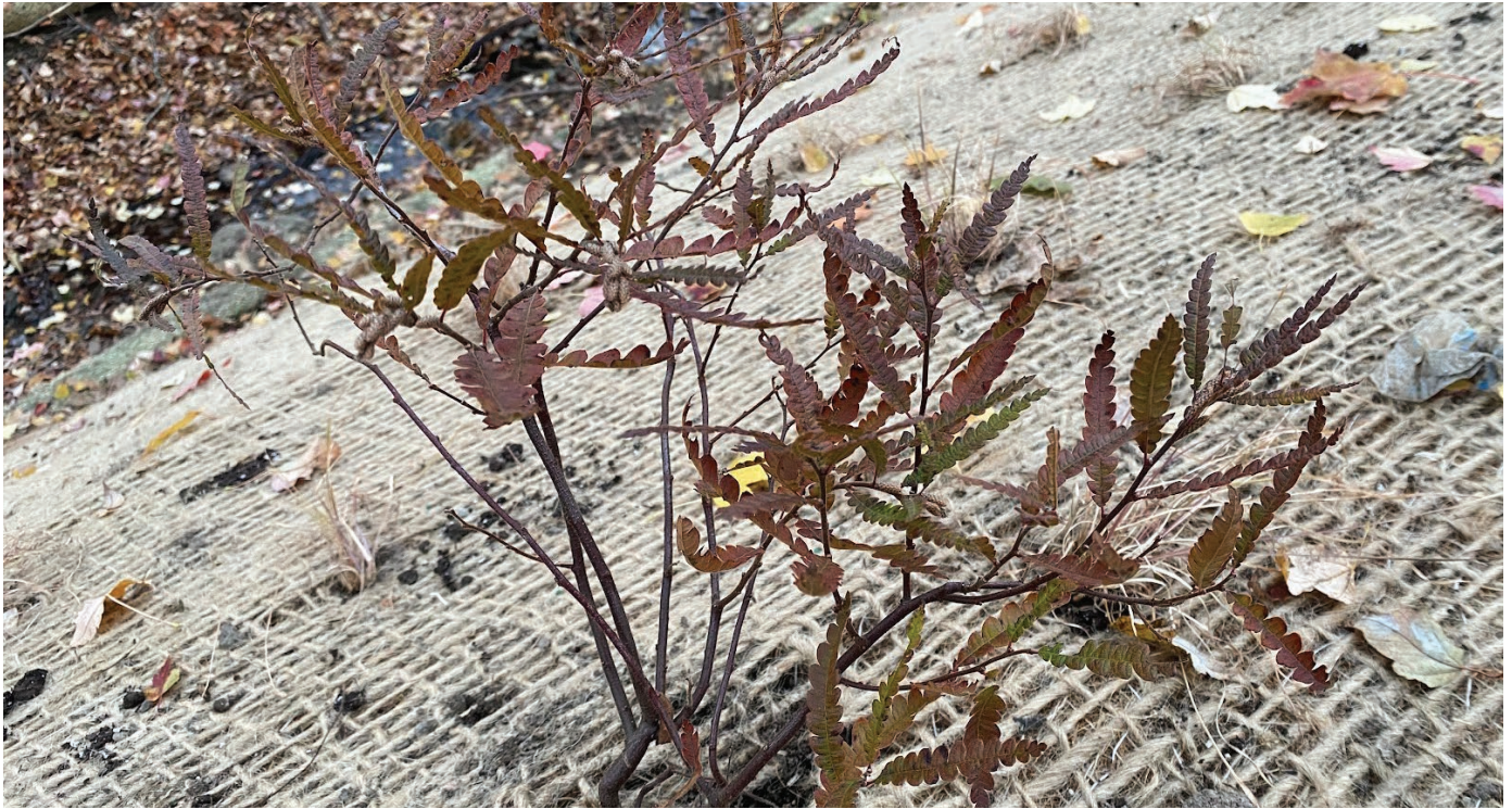
Comptonia peregrina planted at the top of the slope in the erosion control blanket
