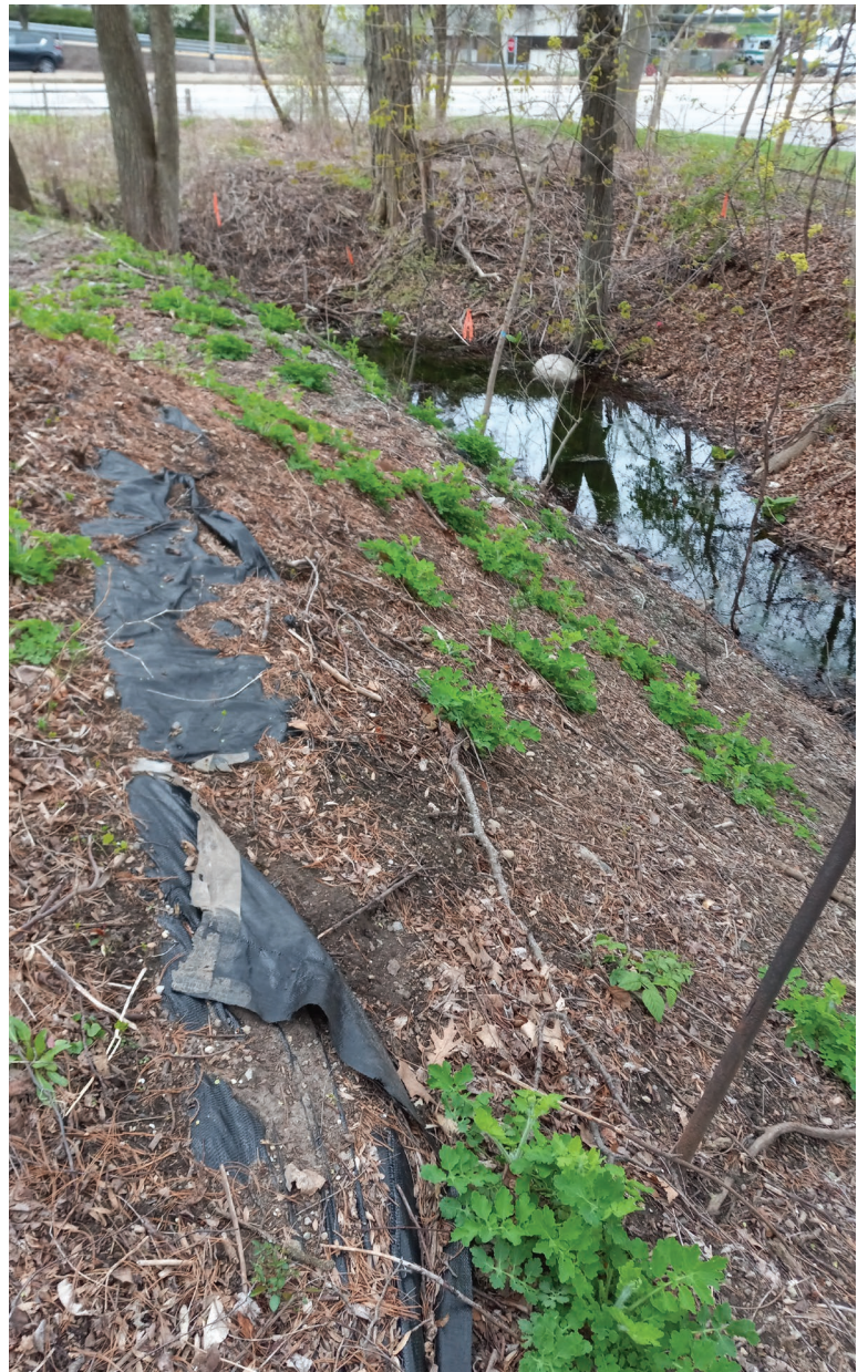
Invasive Greater Celandine (Chelidonium majus) before removal. All silt fence and a large amount of asphalt were also removed
